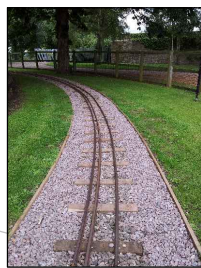
Detail A Typical arrangement of track 1.2m wide ballasted track bed with timber edging each side
